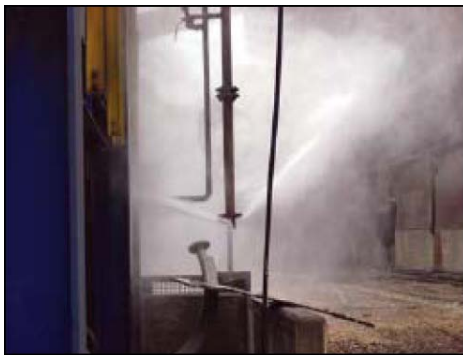
Internal washing of a pipe
