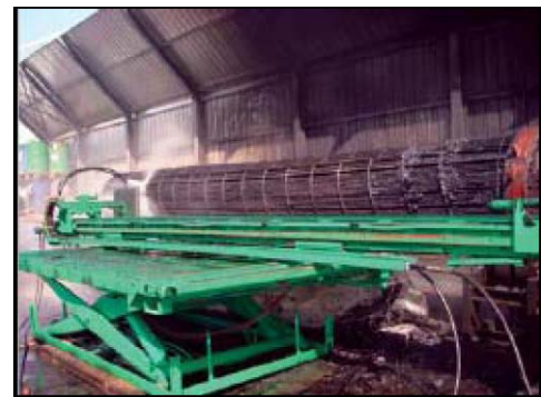
Internal washing of a pipe
