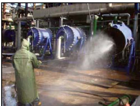
Internal washing of an exchanger with an operator
